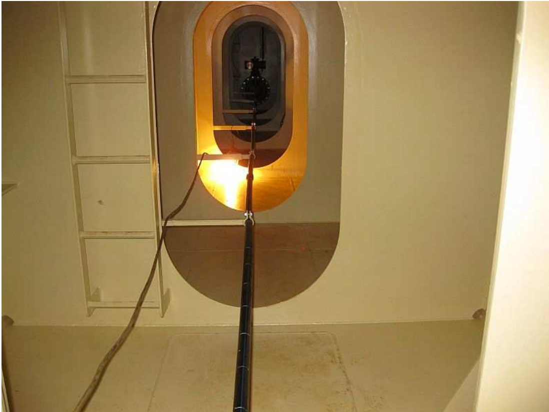
ANTI-EIS-System in einem RO-RO/LO-LO-Schiff
